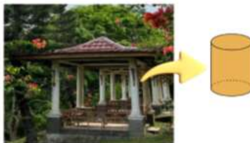
Gambar 3. Tiang Gazebo Bukit Sulap
